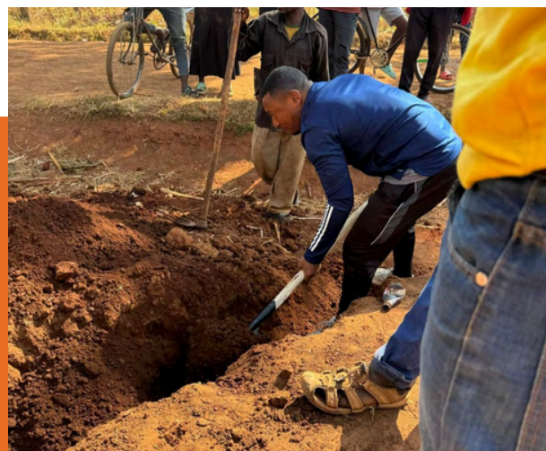
LOCAL VOLUNTEER DIGGING A PATH FOR THE WATER PIPELINE
